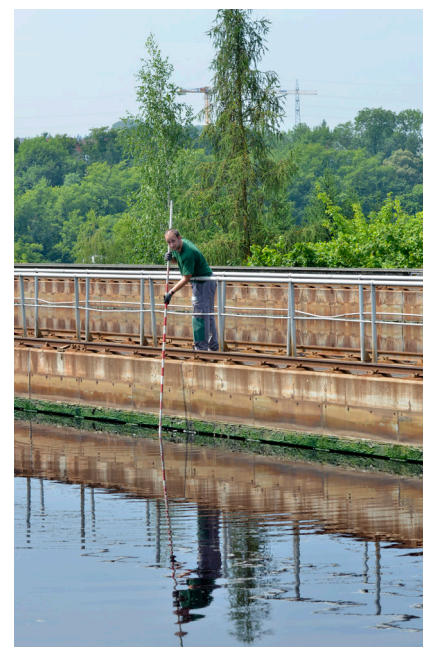
Effluent treatment operative measuring visible depth in the secondary sedimentation basin of the treatment plant.
