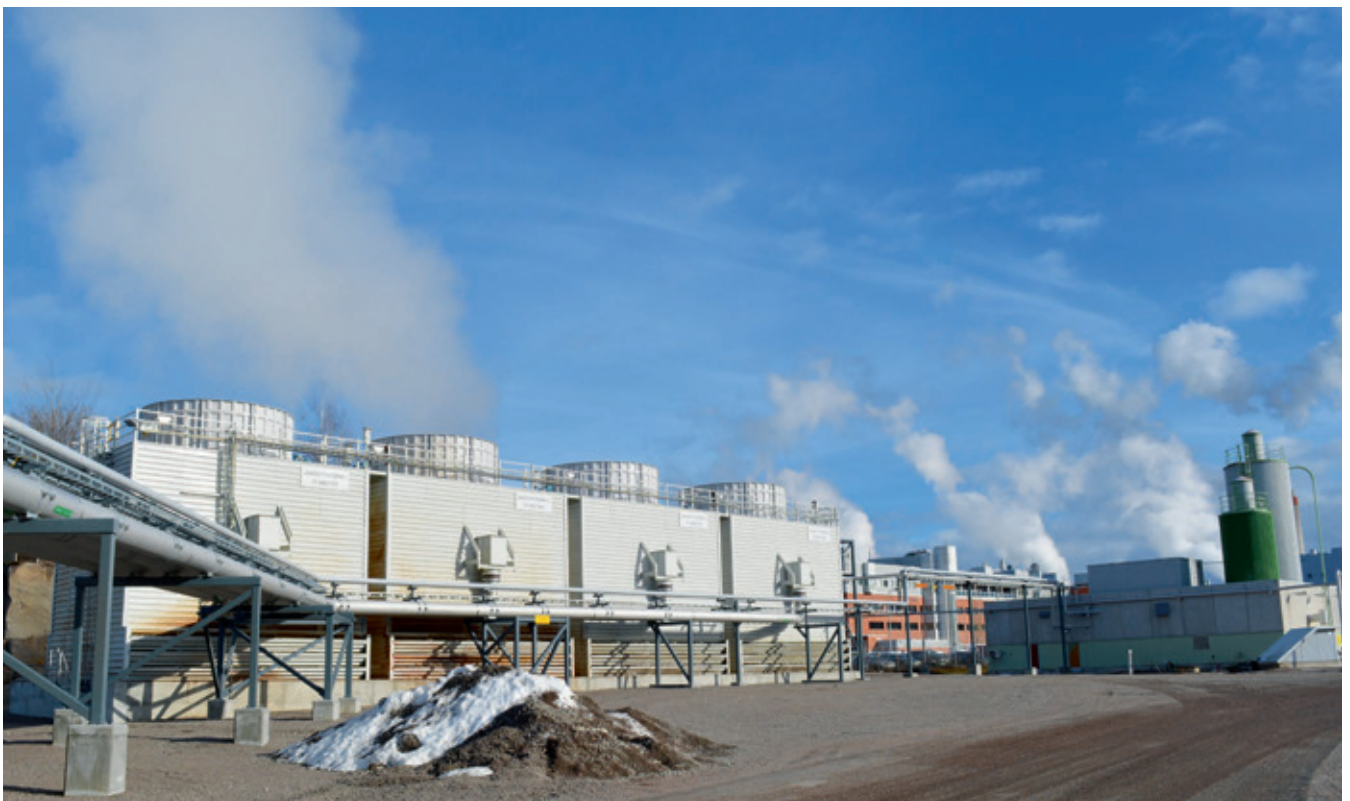
Effluent cooling towers were commissioned in the summer of 2016 to improve the cooling capacity for wastewater, the effluent treatment process and the operational reliability of the effluent treatment plant as a whole.
