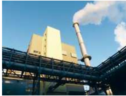
The biomass boiler produces green electricity. This is achieved through the use of biofuels which supply the boiler, and the purification of flue gas.
