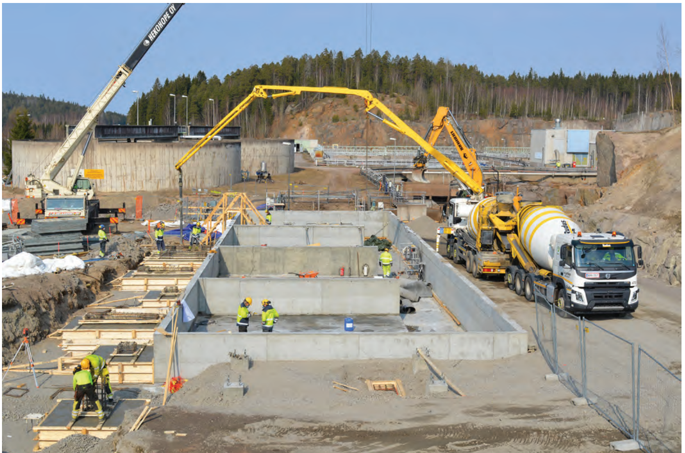
The construction of cooling towers for the biological effluent treatment plant will be completed during the summer. Foundation for the towers was laid in March.
