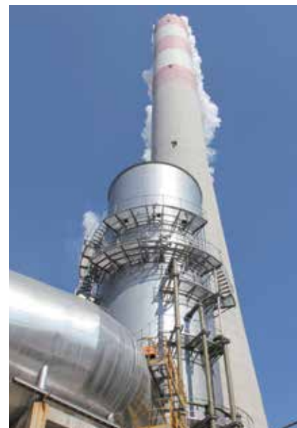
A new flue-gas sulfur dioxide scrubber
