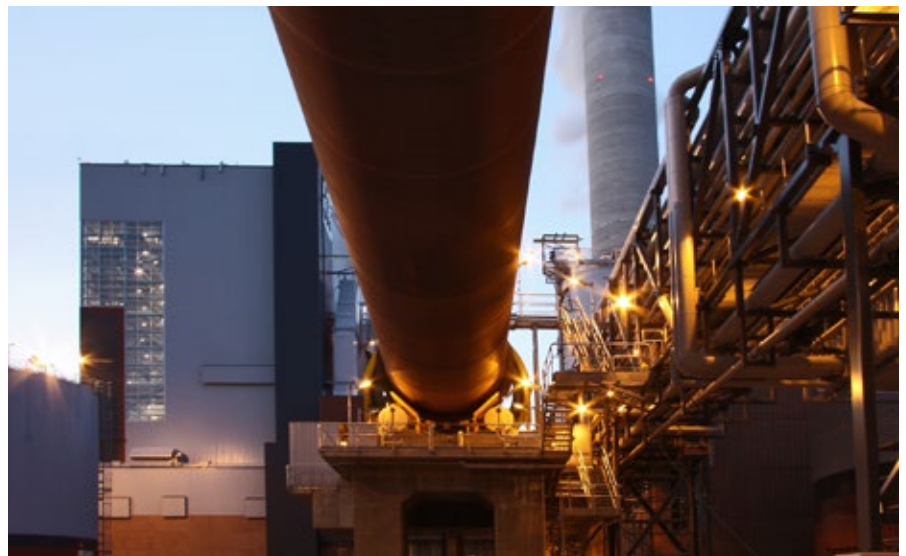
The cylinder-shaped lime kiln in the middle of the picture is an important component of the mill's chemical circulation. The lime kiln's electrostatic precipitator capacity will be increased during the 2021 maintenance shutdown to reduce particle emissions.
