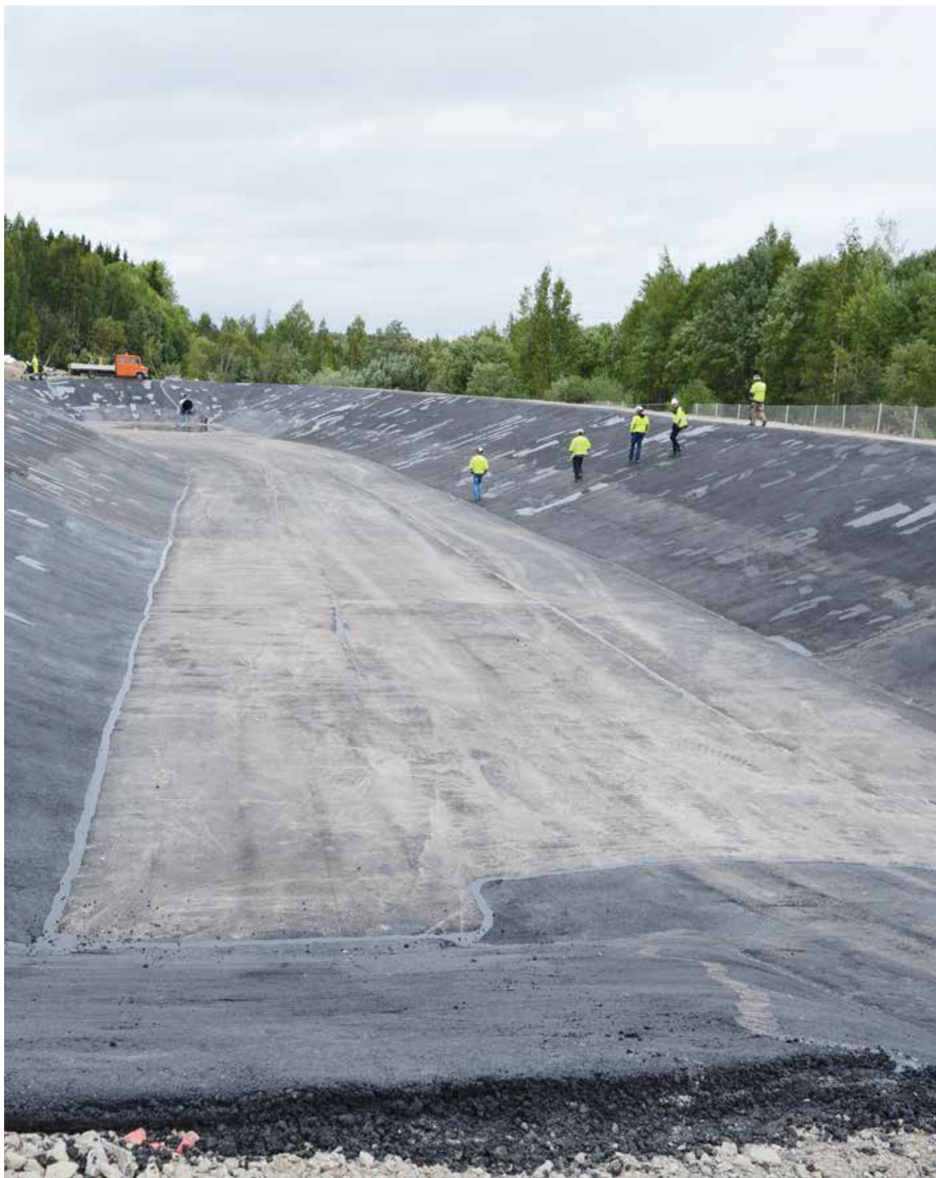
The stormwater detention basin completed in 2018 ensures that the solids present in stormwater runoff, such as fine particles from wood and bark, remain in the basin. This sedimentation basin reduces the nutrient load of the Kymijoki river. The basin is 140 metres long and 30 metres wide, and its depth varies from 3 to 4 metres. The volume of the basin is approximately 5000 cubic metres.
