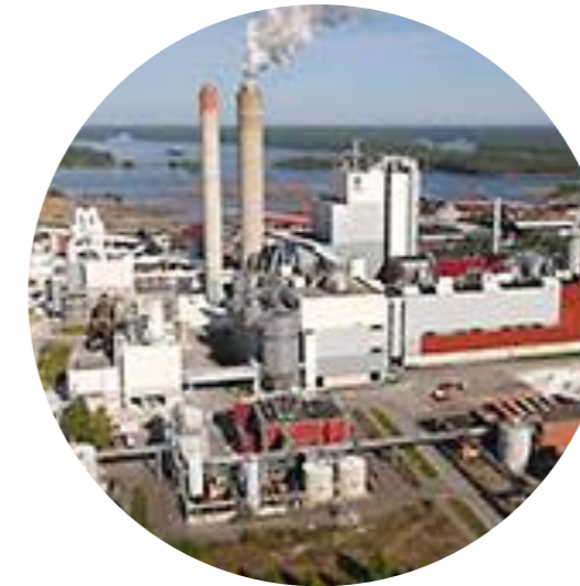
Kaukas pulp mill efficiency improvement, paper and pulp decoupling completed
